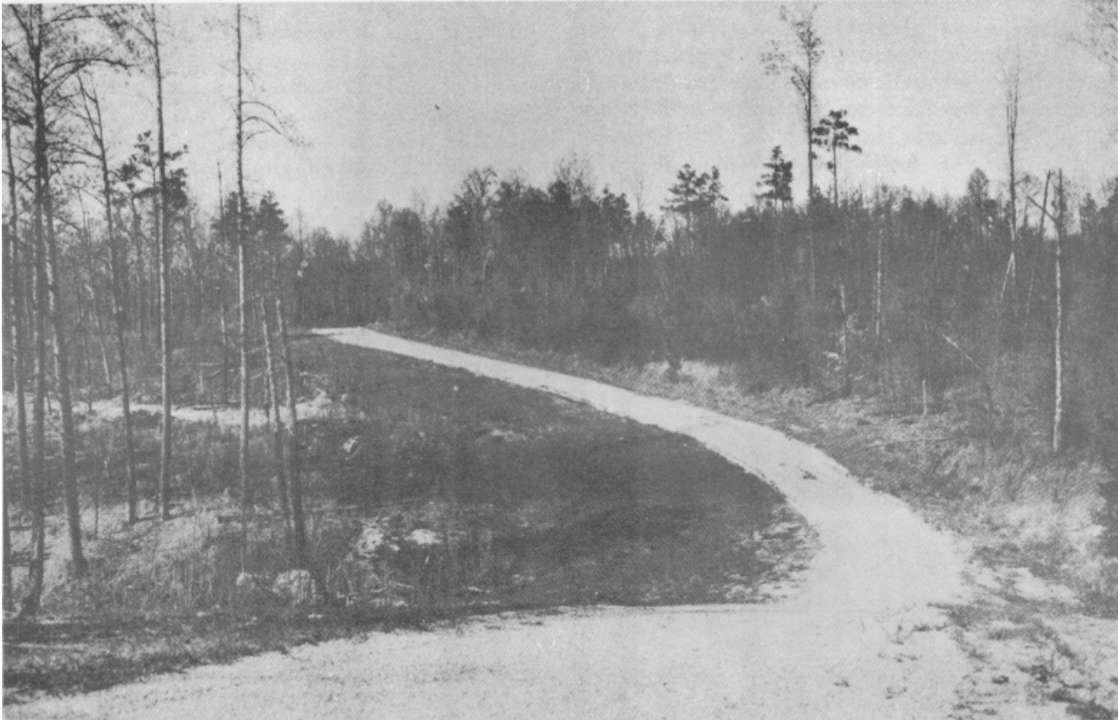
Figure 10-12. Vegetated firebreak with rock-surfaced patrol road
